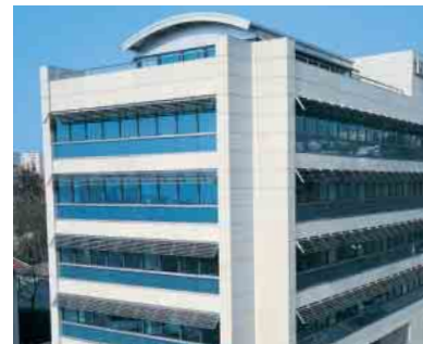
Enka Building, Стамбул, Турция Enka Building, Istanbul, Turkey
